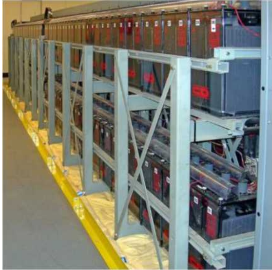
Accumulator batteries of the backup power source of the data center.
